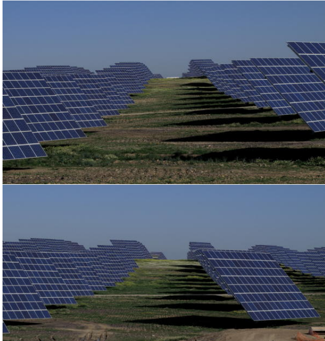
Figure 1: Two general views of the array of PV panel assemblies.
