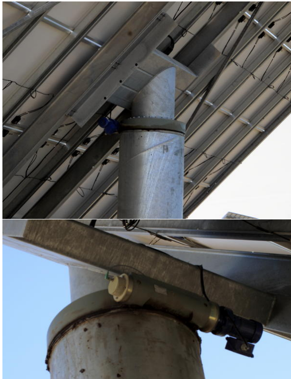
Figure 2: Drive mechanics for a panel assembly. The drive consists of a fixed ring gear mounted on the support post and a motor driven worm gear.
