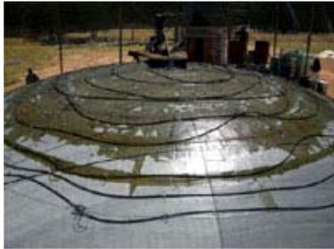
**Figure 28.** Transferring the dish resin
