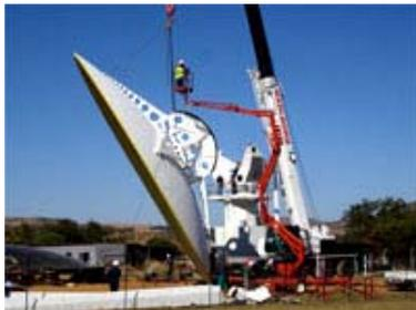
**Figure 29.** Lifting the dish onto the pedestal; followed by installation of the feed support legs
