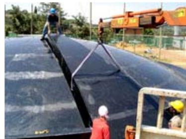
**Figure 24.** Placing the last segment of the dish mould
