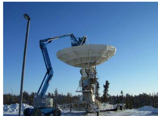
**Figure 8.** The MV-1 antenna being disassembled in -30C conditions in Yellowknife. At least it was sunny!
