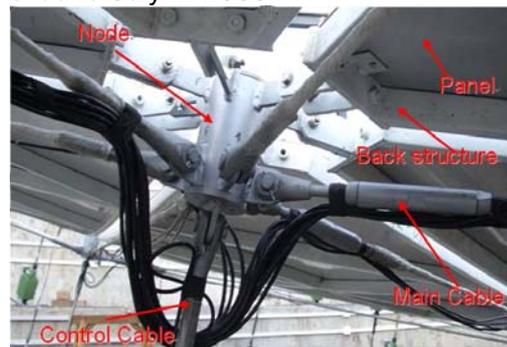
Fig.4. Structure of cable-mesh Reflector
