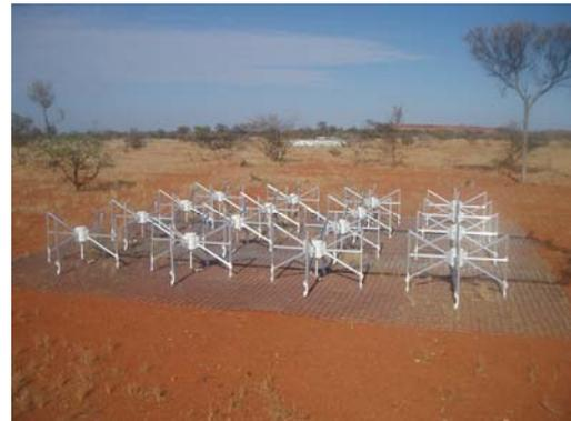
**Figure 3.** An MWA tile in the field, showing the ground-plane and the 16 dipoles. Credit: Steven Tingay
