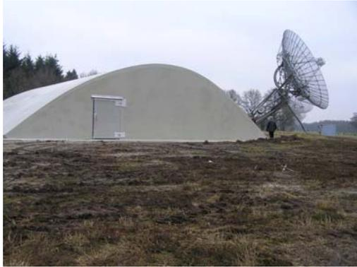
**Figure 13.** The new radome at Westerbork is setup between antennas 4 & 5 of the WSRT. It covers an area of over 160 sq. metres. There will be a 12x12 tile aperture array setup inside, with the first tiles to be installed in January 2009
