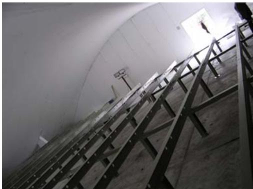
**Figure 14.** Inside the radome, beams of composite material are used to make the platform for the tiles European Plans after the end of SKADS
