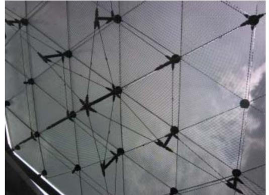
*Figure 1. Segment of pre-stressed, reflector back-up structure.*
