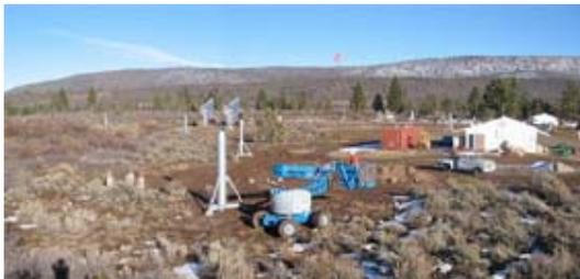
*Progress at the ATA site where 32 antenna pedestals have already been completed and the dishes will be installed early in the new year.*
