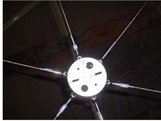
*Fig2b FAST cable-mesh reflector: node structure*
