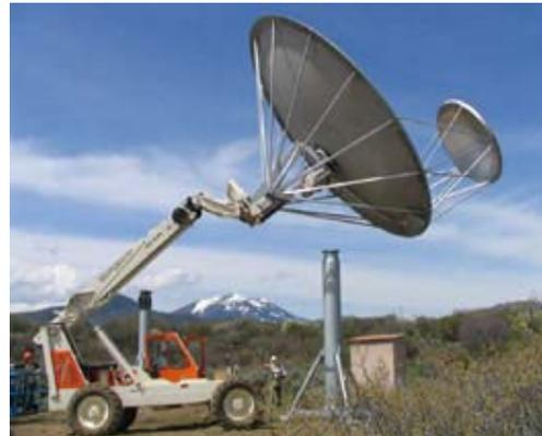
*An ATA antenna being emplaced. The pedestals with the underground infrastructure are installed first; then the remainder of the antenna is assembled in the construction tent and emplaced as a unit. The antennas and mounts arrive on-site as “kits,” which may be assembled and installed in just a few days by a small staff.*
