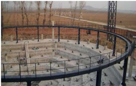
*The wiring network around the depression for signal and power supply to the main reflector, the measurement and control components, together with the cable-car to mount the focus cabin supported with cables to the towers.*
