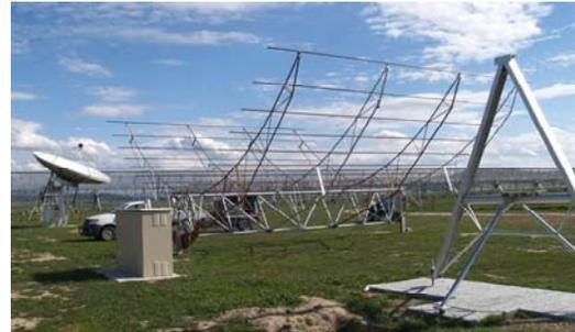
*Meshing of the Rapid Prototype Telescope for the SKA Molonglo Prototype*
