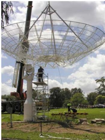
*The dish of one of the NTD antennas being lifted onto its pedestal*
