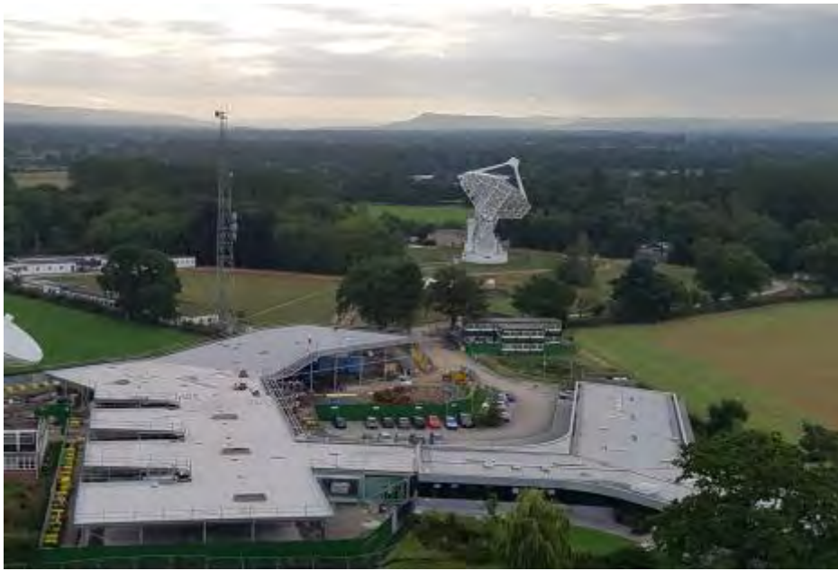
Construction of new HQ extension continues
