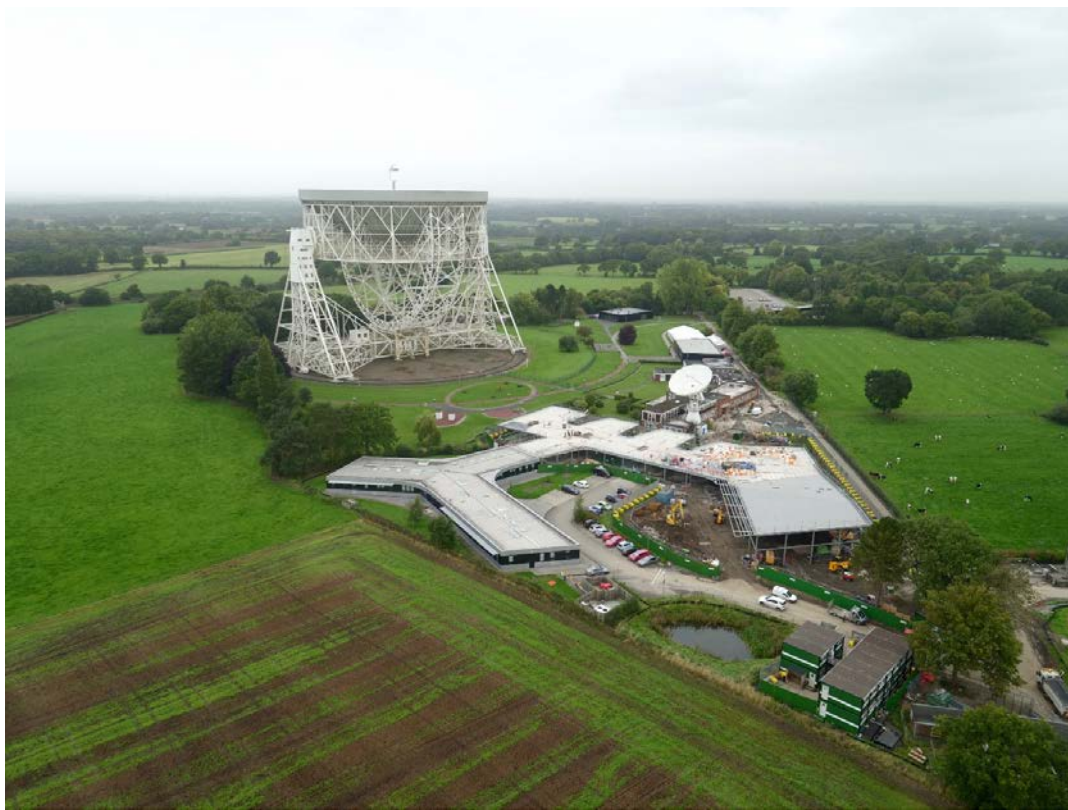
Construction of new HQ extension continues
